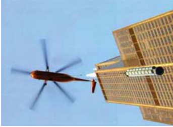
A helicopter was used to lift an antenna to the top of the Sears Tower. Photo courtesy Radio Frequency Systems.
